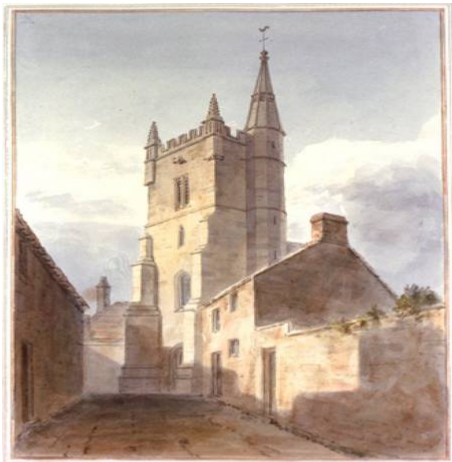
1804 by John Buckler from south under the directions of Colt Hoare
